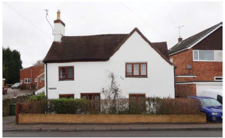
Fern Cottage on Main Road
