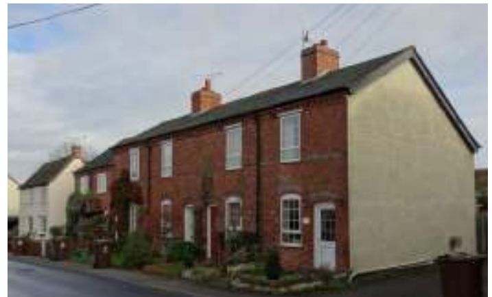
Terraced properties located on Windmill Lane
