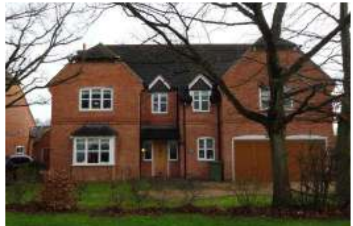
New build dwelling set back from Kenilworth Road
