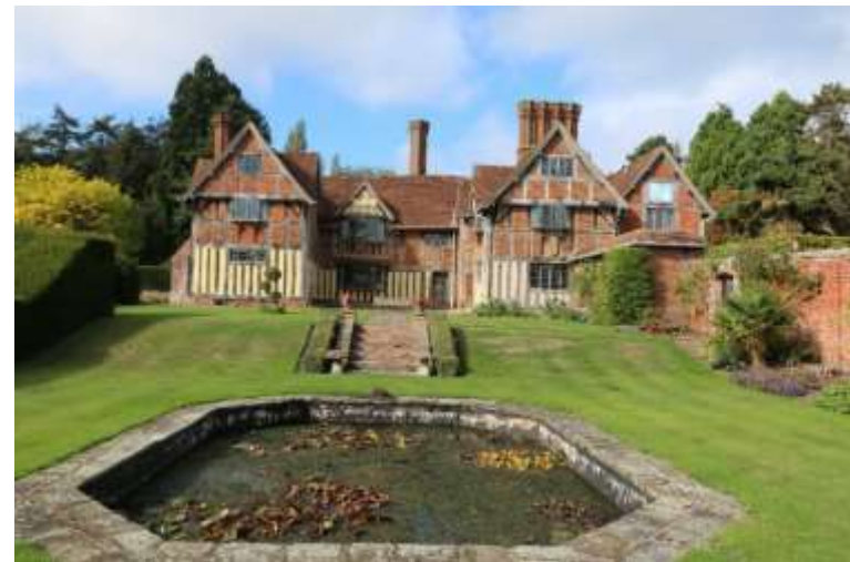
Figure 8 Grimshaw Hall; east rear elevation
