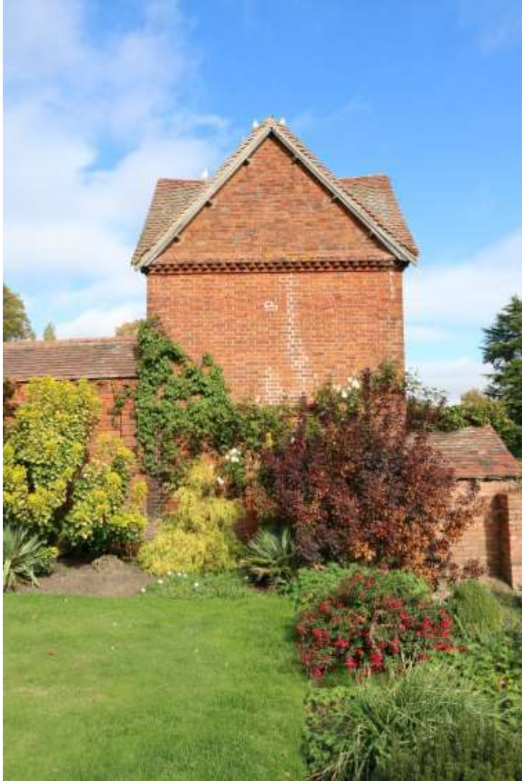
Figure 9 Grimshaw Hall; dovecote east of hall
