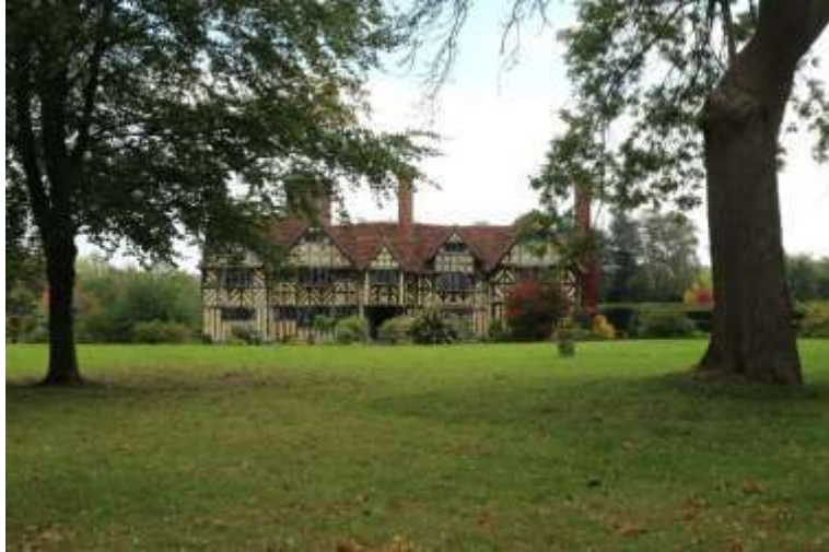
Figure 24 front elevation of Grimshaw Hall from lawns/parkland adjacent to Hampton Road
