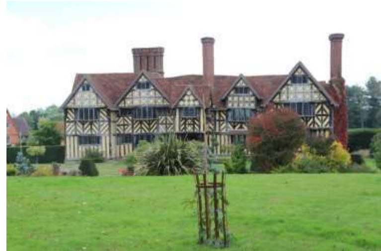
Figure 7 Grimshaw Hall; west front elevation
