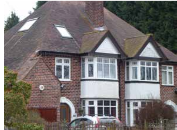
Photo : Typical Tidbury Green Residential Vernacular
