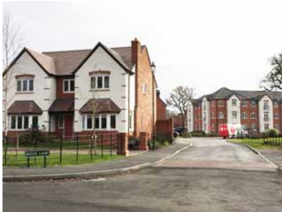
Photo : Typical Dickens Heath Residential Vernacular
