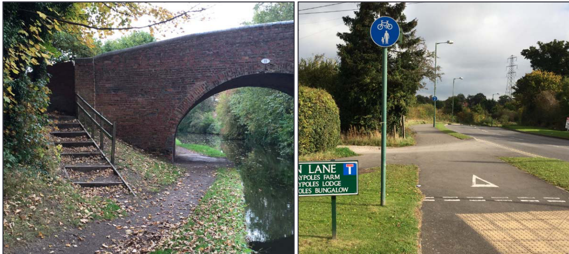
Stepped Access from Canal to Tythe Barn Lane
