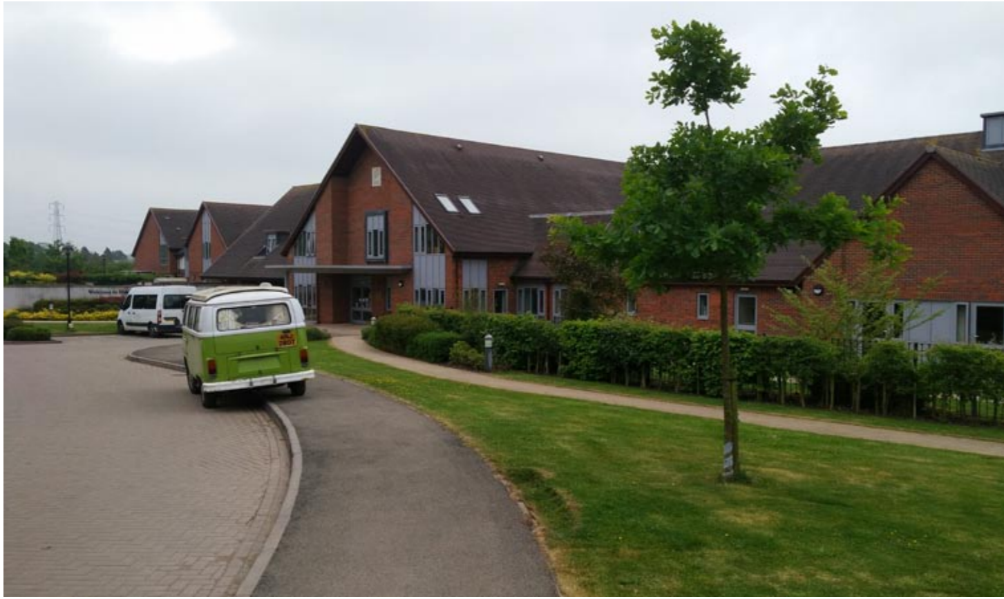
Photo P9 - Harper Fields Care Home which abuts the western boundary of the proposed allocation site
