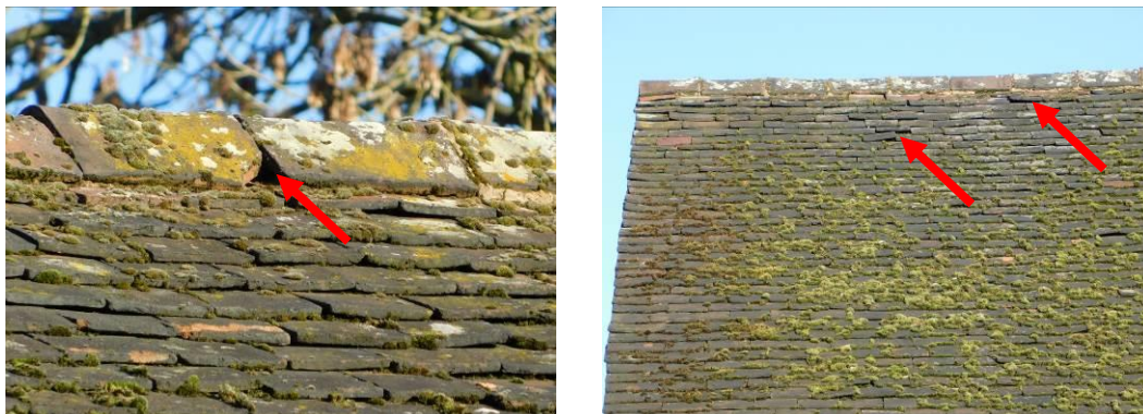
Figs. 23 & 24 Ridge and roof tiles
