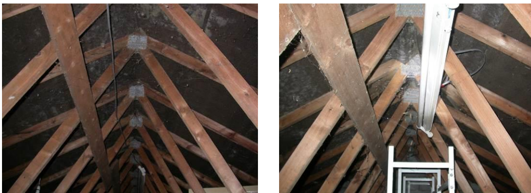
Figs. 31 & 32 Trussed rafter roof void
