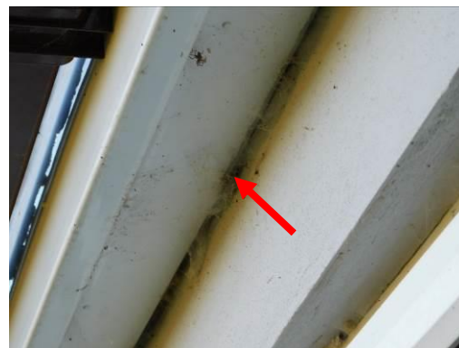
Figs. 29 & 30 Eaves soffit gap
