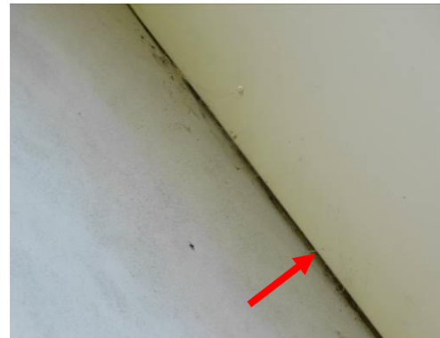
Figs. 27 & 28 Gaps along gable soffits
