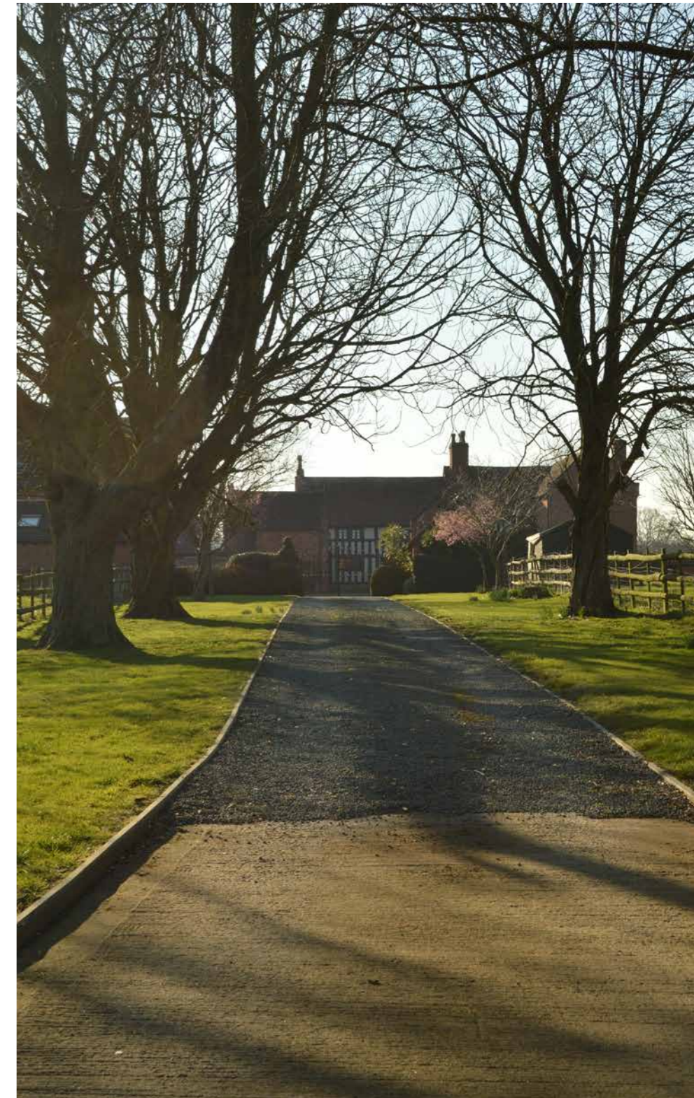
Looking west to the Jerrings Hall complex from Tanworth Road
