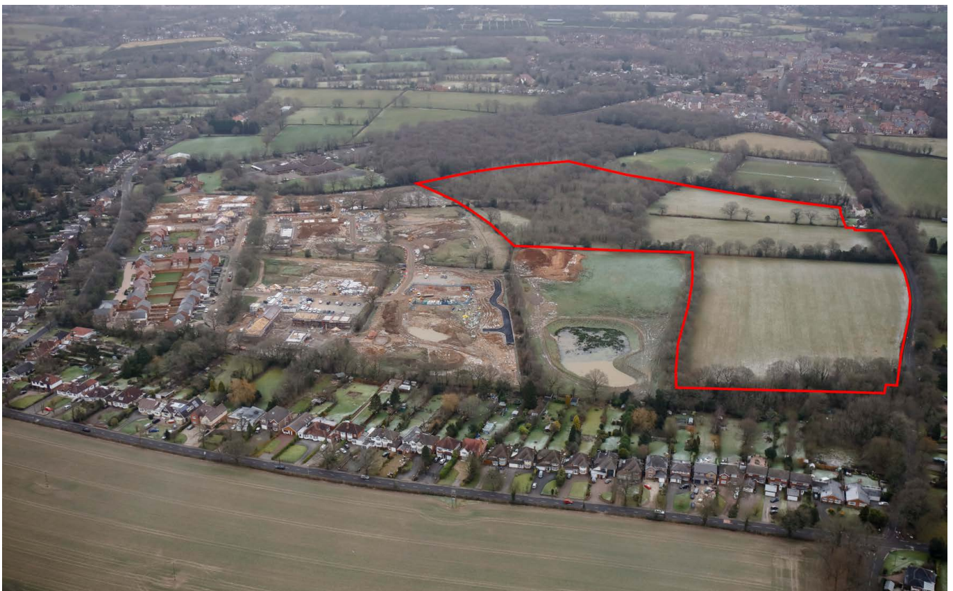
Figure 1. Bird's Eye View of Site looking north (land to left is Bellway Homes scheme under construction)
