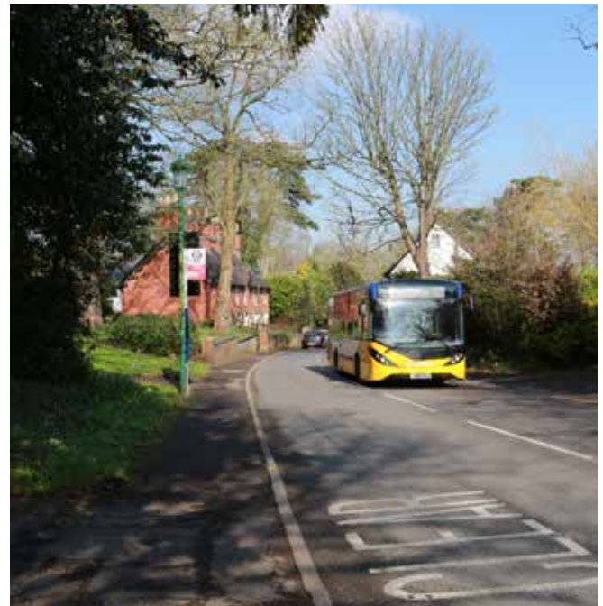
Bus stop along the High Street (B4102)
