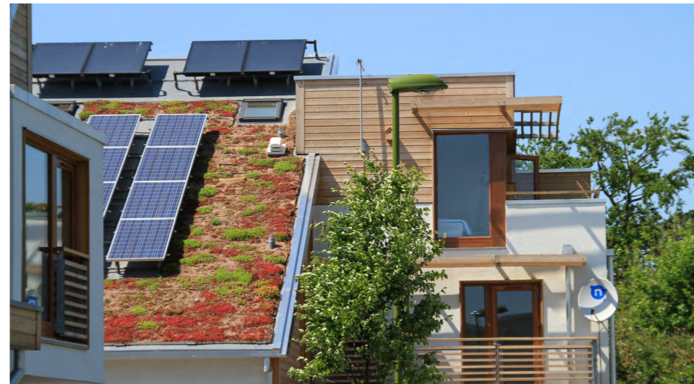
Example of PV panels integrated into roofscape
